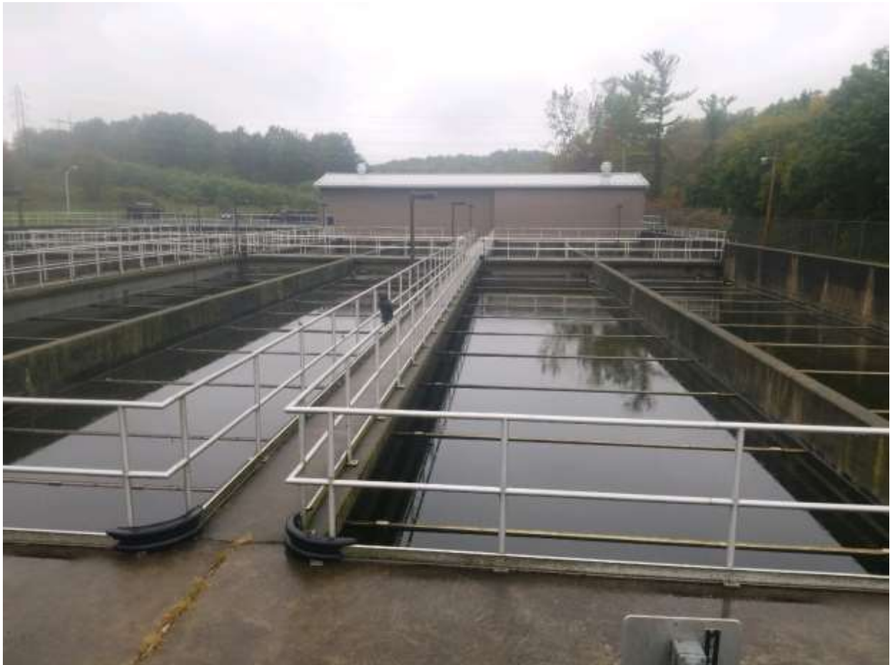
Figure 1 - UV Disinfection Building at the end of the Final Tanks.
