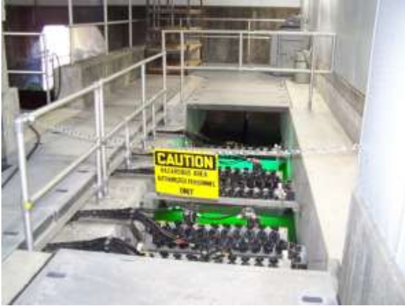
Figure 2 – UV disinfection modules and UV bulbs.
