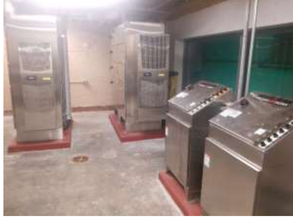
Figure 3 – UV disinfection control room.
